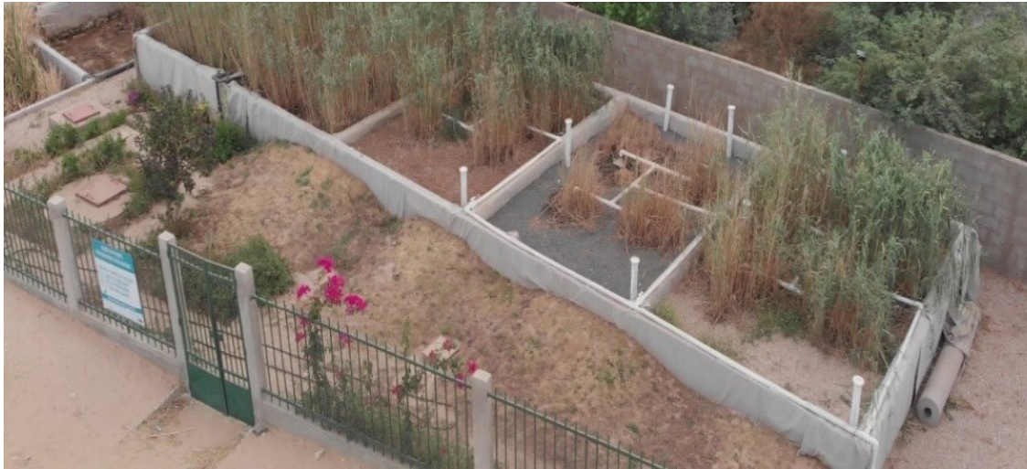
Ecological wastewater treatment plant (Saint Louis, USA)
