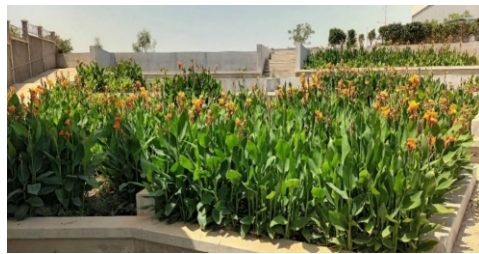
Surya Varsani Academy, Bhuj, Gujarat (0.12 MLD)
