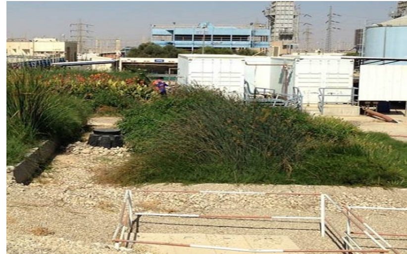
Ramat Hovav, power station, Israel Constructed Wetland
